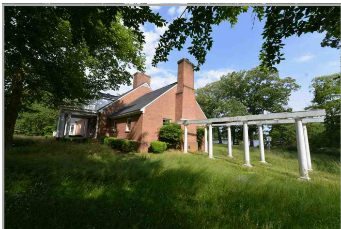
View of pergola on east side of residence.
