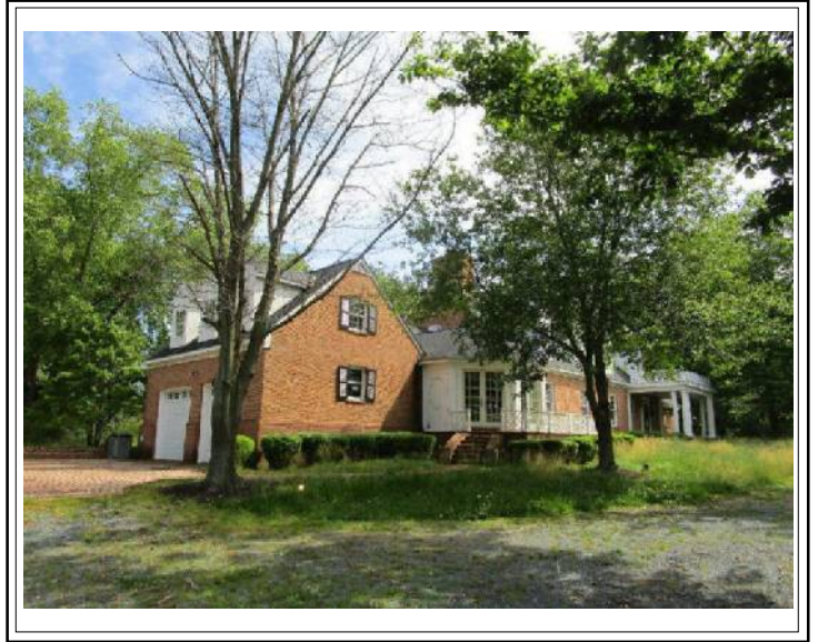
Additional Front Photo #1
