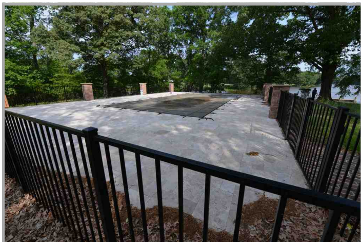
800 sf. in ground concrete waterside swimming pool with slate tile apron.
