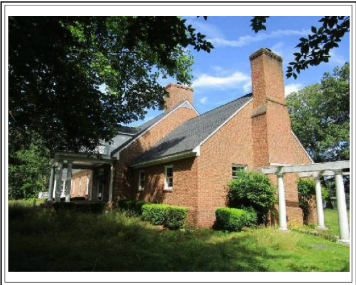
Additional Front Photo #2
