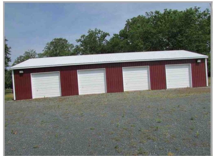
30 x 72 four bay out building of all metal construction.
