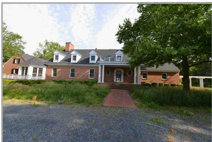
Front view of Subject residence. All brick construction with covered porch supported by columns.
