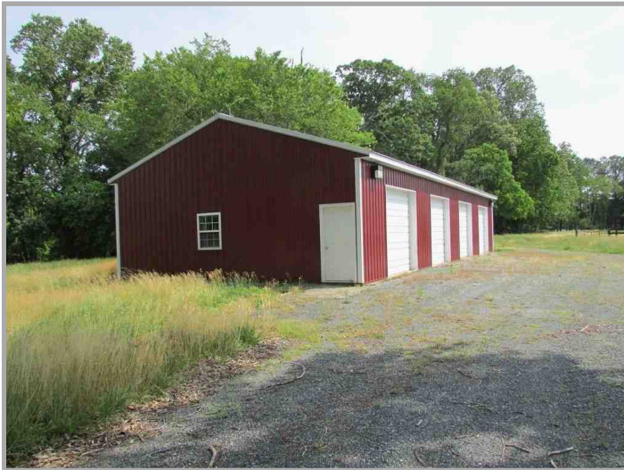
Out building is in good condition and well maintained.
