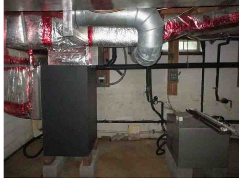
Geothermal Unit
