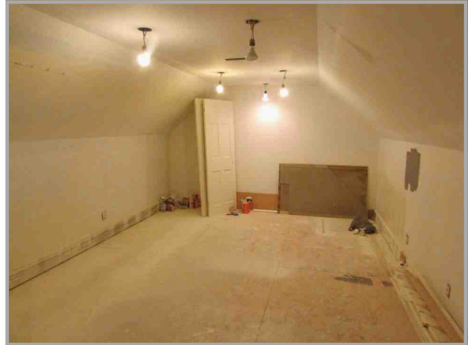
Unfinished second floor bedroom.
