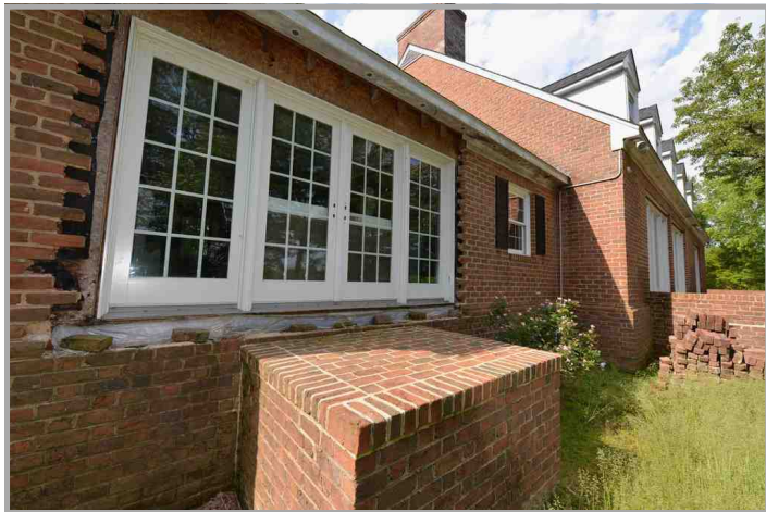
View of unfinished brick work around French doors in master bedroom.
