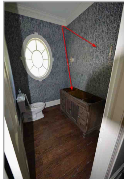
Half bath off foyer. Half bay shows missing sink and mirror.
