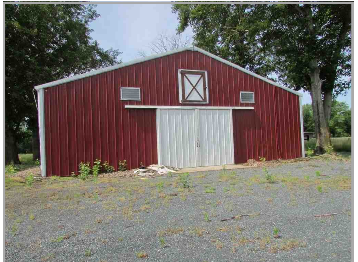
Front of horse stable with sliding barn door. Building in good condition and well maintained.
