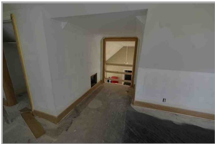
View of wall cut out.
