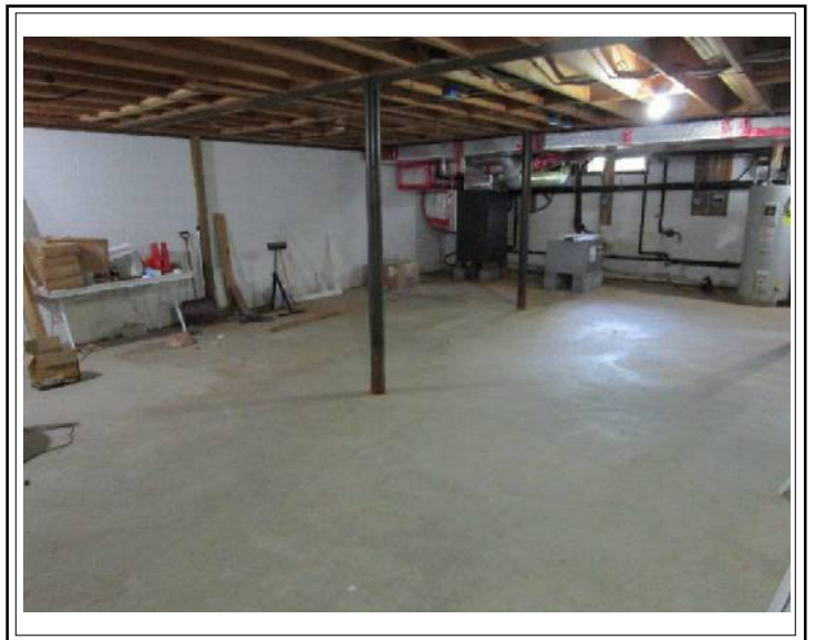
Basement - Unfinished Area
