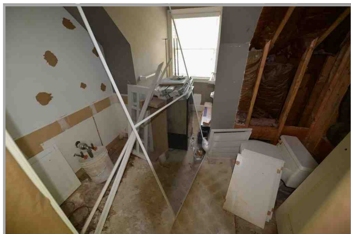
View of bathroom under construction.
