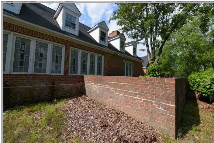
View of raised brick patio at the rear.
