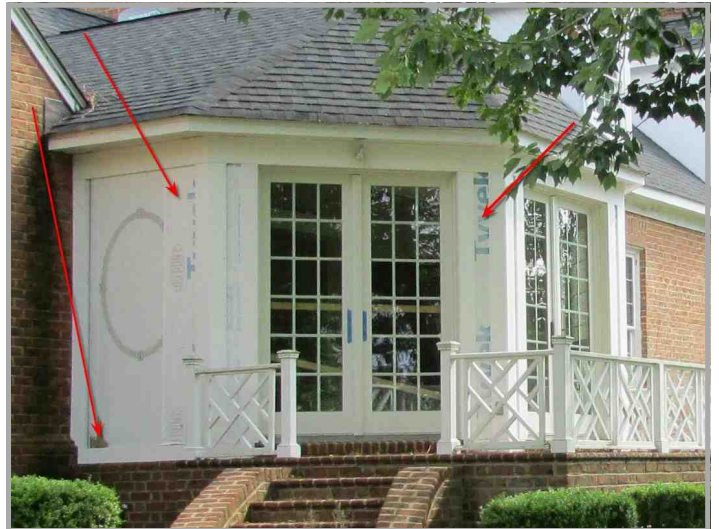
Exterior of breezeway shows unfinished new construction.
