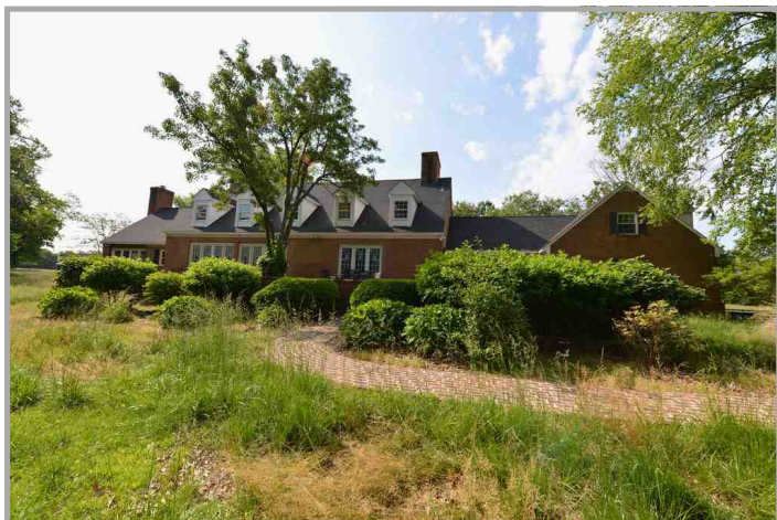
North profile shows overgrown landscaping.
